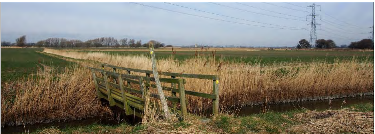
Fig. 46: Bridge over Tore Petty Sewer, near Midley Church
