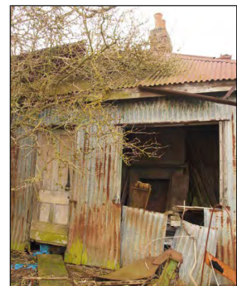
Fig. 58: Looker's hut at Buss Barn. The fireplace can be seen in situ through the window.
