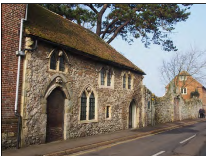
Fig. 64: Medieval buildings in New Romney
